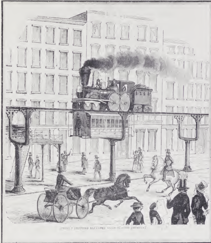
A proposed elevated railway for Broadway (1850), with passenger coach beneath the locomotive. (Parsons' Print Collection)
